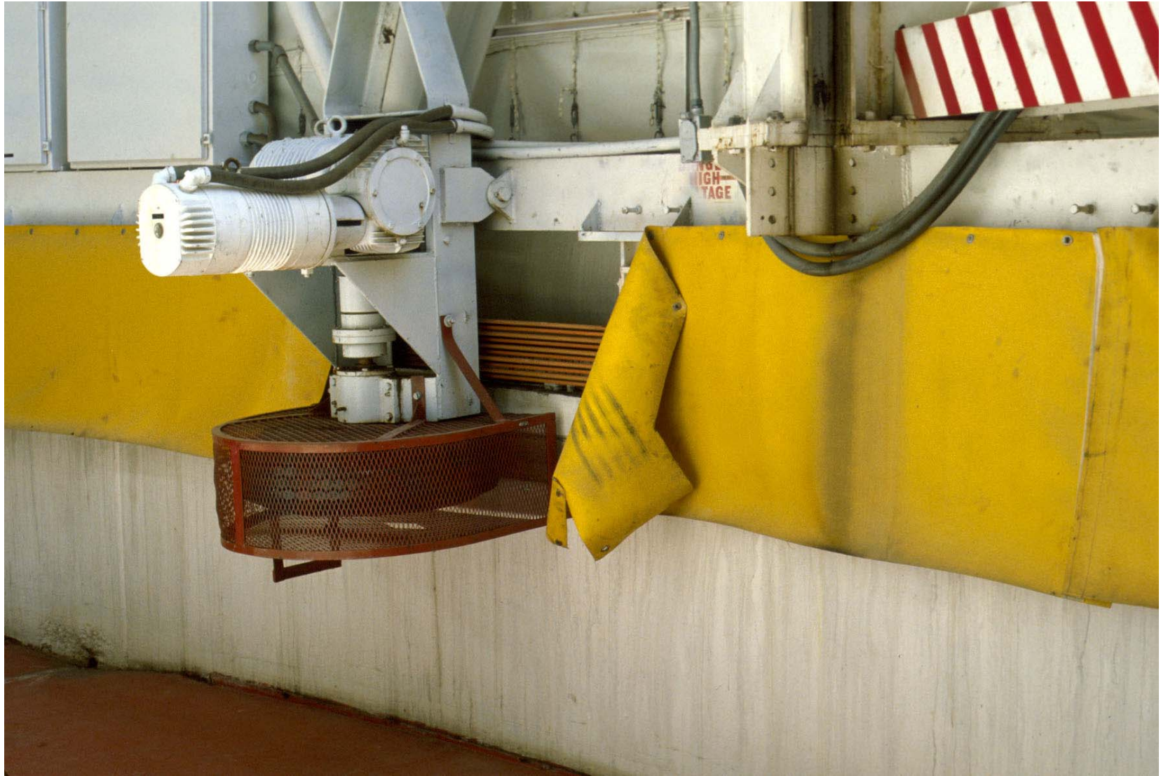
One of four variable speed azimuth drives for astrodome
